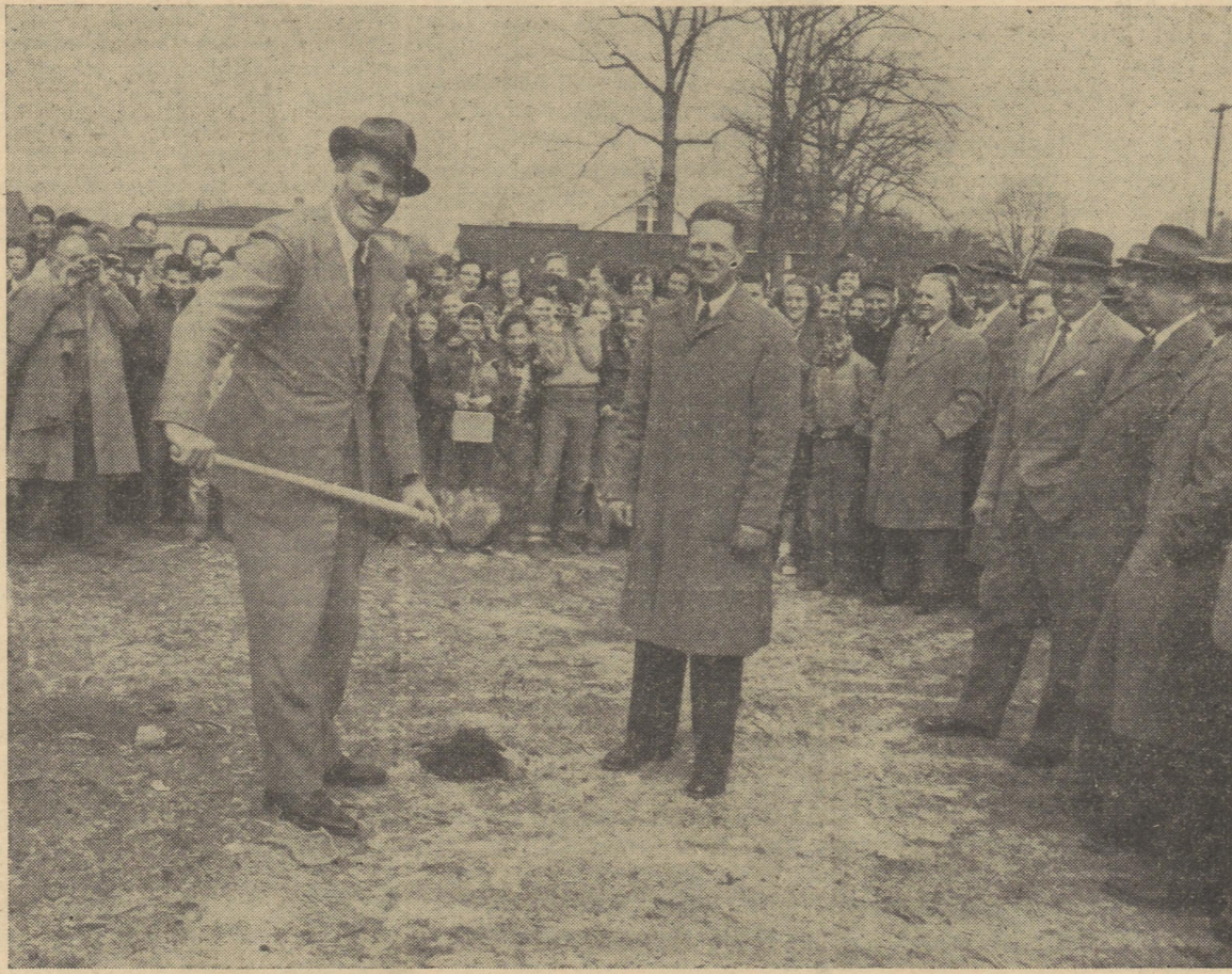
Gov. Elbert N. Carvel digs up the dirt in a ceremony Friday afternoon in which ground was broken for Harrington's new elementary-school building. Standing by is Robert Nelson, president of the Board of Education.
