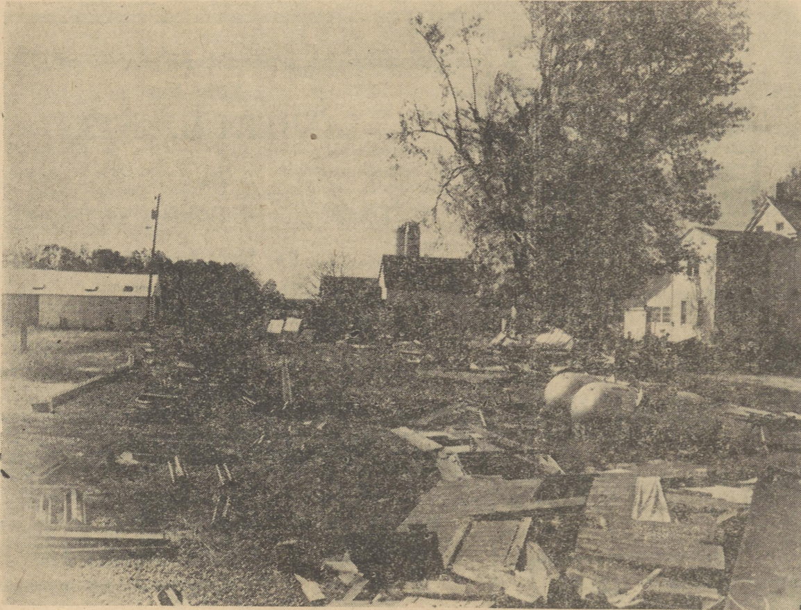
Broiler Houses Leveled by Wind
