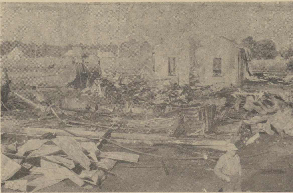
AFTER THE FIRE WAS OVER—Looking east, one sees the ruins of the R. W. Vane cannery after it was destroyed by fire Friday afternoon.—Curtis Melvin photo
