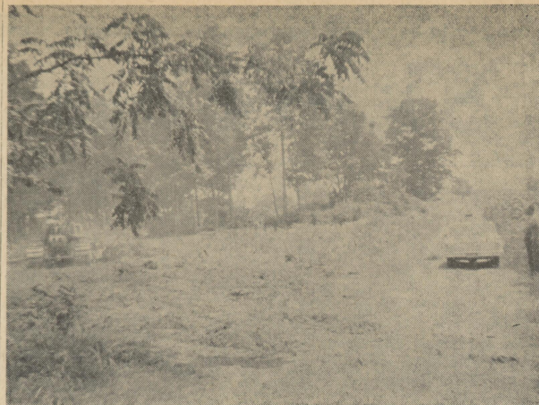
THE NINTH GREEN — Of the Garrison Lake Country Club, to be ready in May of next year between Smyrna and Dover on U. S. 13. Construction is underway. Mr. and Mrs. Charles Ewing are the owners.
