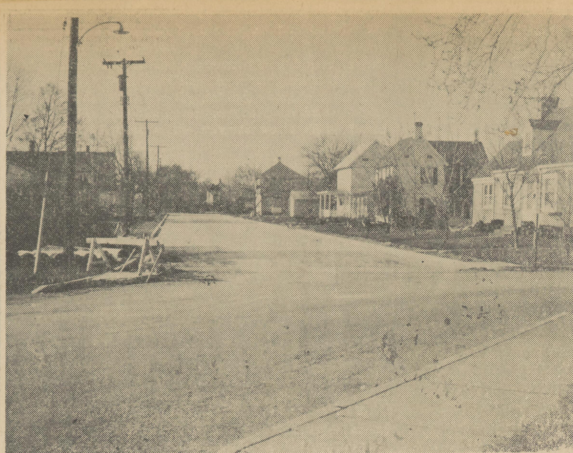
SECOND STREET HAS A NEW LOOK NOW, with improvement being done by Paul Scotton Construction Company, Dover. The street has been curbed and blacktopped, with final coat expected next spring. Installation of sidewalks may be completed this week, depending on the weather. Price photo
