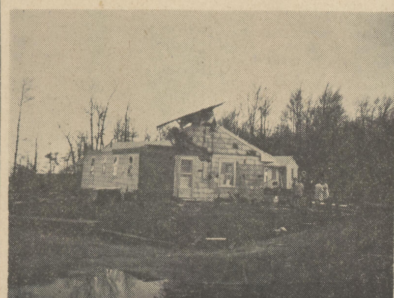
HOW FIRM A FOUNDATION — Did not apply to this residence of Mr. and Mrs. Richard Adams, of Felton Manor, destroyed by a tornado Friday afternoon. It was moved from its foundation. — Price photo
