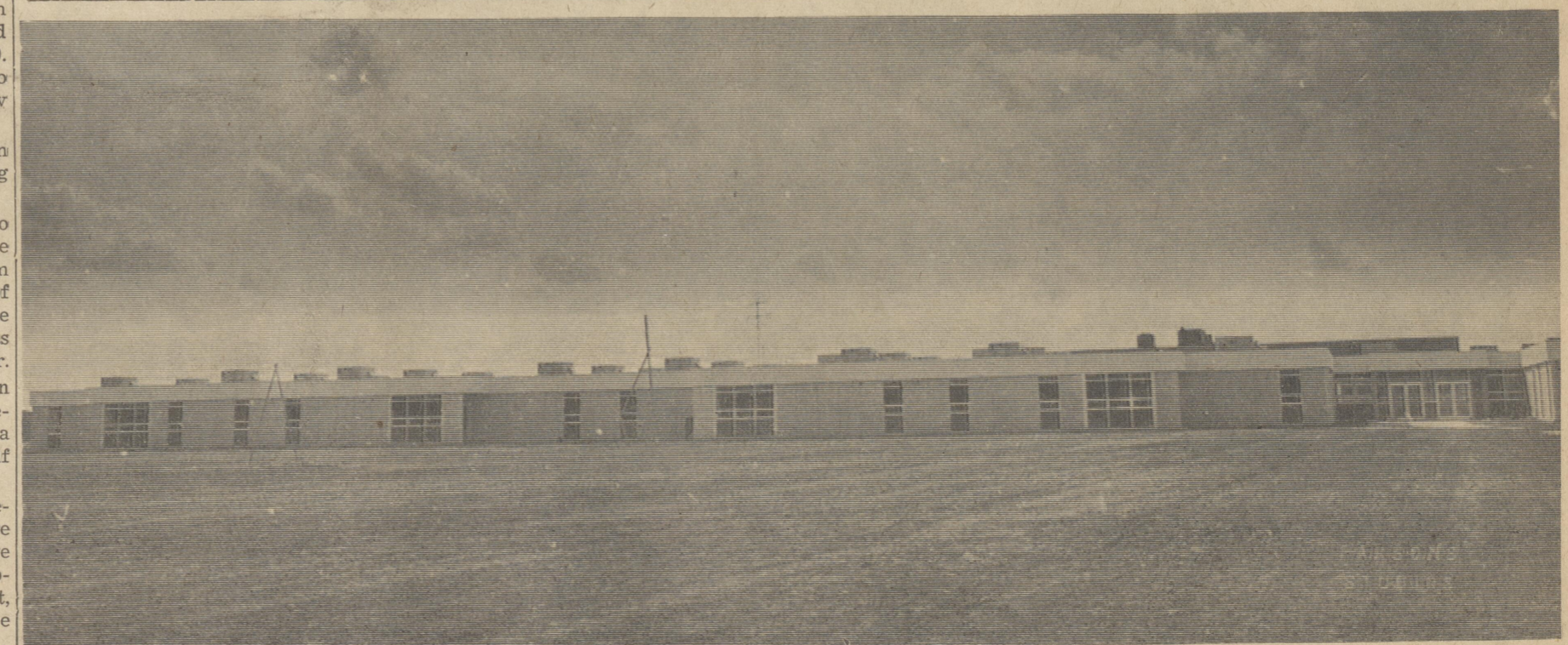
LAKE FOREST HIGH SCHOOL — The new school held its first classes Wednesday. The structure, not completed, has sufficient classrooms to operate. High-school pupils from Harrington, Felton, and Frederica, attend the school near Killen's Pond. Parsons Studio photo
