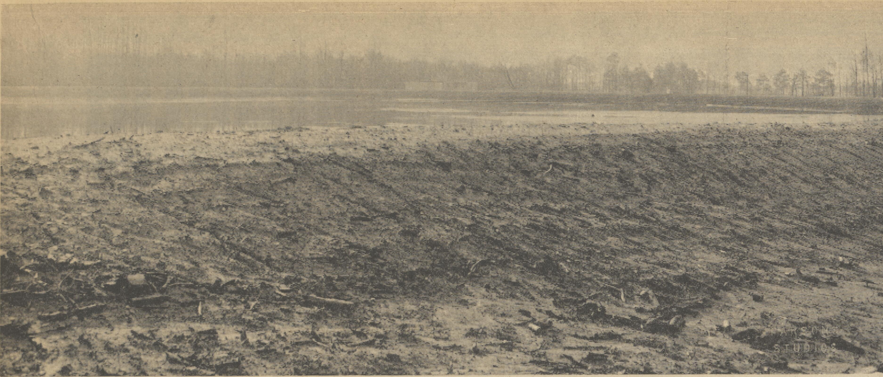
SCENE OF FULL-TIME ACTIVITY — This is one of two polishing ponds at Harrington's new sewage-disposal plants. Monday night, the City Council told Dale Phillippi, to start Tuesday working full-time to manage the plant and to make improvements. This is necessary to qualify for further federal grants. Parsons Studio.
