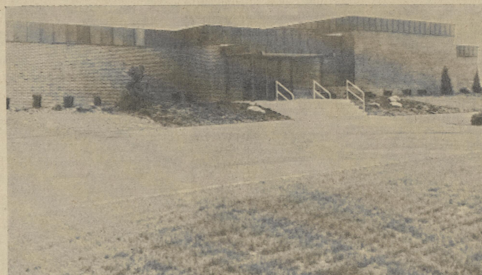
ADMINISTRATIVE FACILITIES OF KENT COUNTY wastewater facilities dedicated Saturday morning near Frederica.
