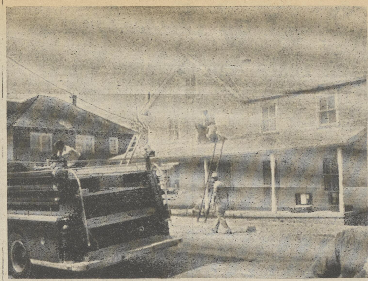
Donald McKnatt selects equipment as firemen on the porch roof remove furniture and Al Mann approaches scene of fire.
