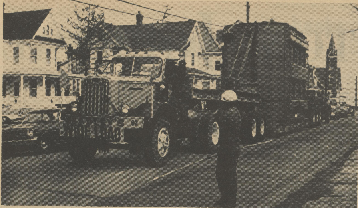
Delmarva Power and Light Co. moved a 100 ton transformer through Harrington last Friday to Denton, Md. The huge transformer which was transported by rail to Harrington, the nearest place to Denton, was moved on the last leg of its journey by truck. It was to be installed at the Steele substation, according to a DP&L official, and will be part of a project of the lower shore area to increase the available energy.
