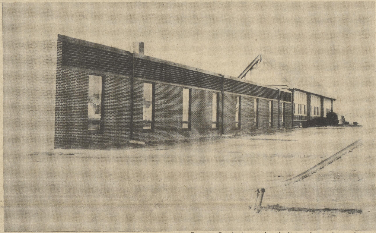
The newly completed wing of Lake Forest Elementary East at Frederica to be dedicated at a later date.
