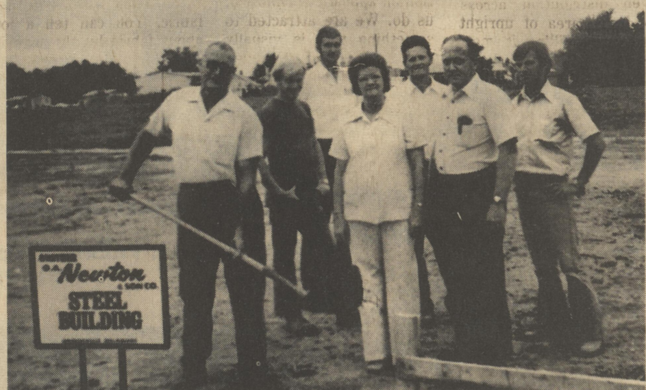
Walter and Marie Messick broke ground last week for a museum on the Taylor & Messick land. O. A. Newton and Son Co. will build the 40' x 115' structure. Standing to Mrs. Messick's left is Mr. Ray Ellerman of Bridgeville, building salesman for Newton.
