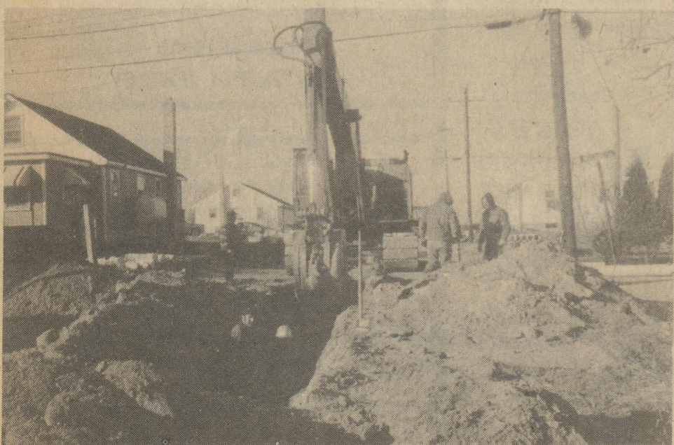
Construction Work Continues.....
