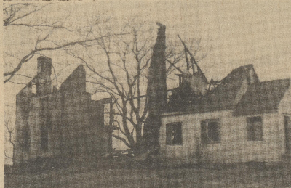
Fire destroyed this very old brick and frame dwelling located just beyond Prospect Church on Rt # 14 west of Harrington. The farm was known as the Raughley Farm, and it is believed that the brick section, being the oldest section, was built in the mid-1700's. The bricks were brought over from England. The Harrington Fire Co. was summoned to the scene on Thursday night but before the house was beyond saving. The Fire Marshall's Office in Dover has the matter still under investigation.
