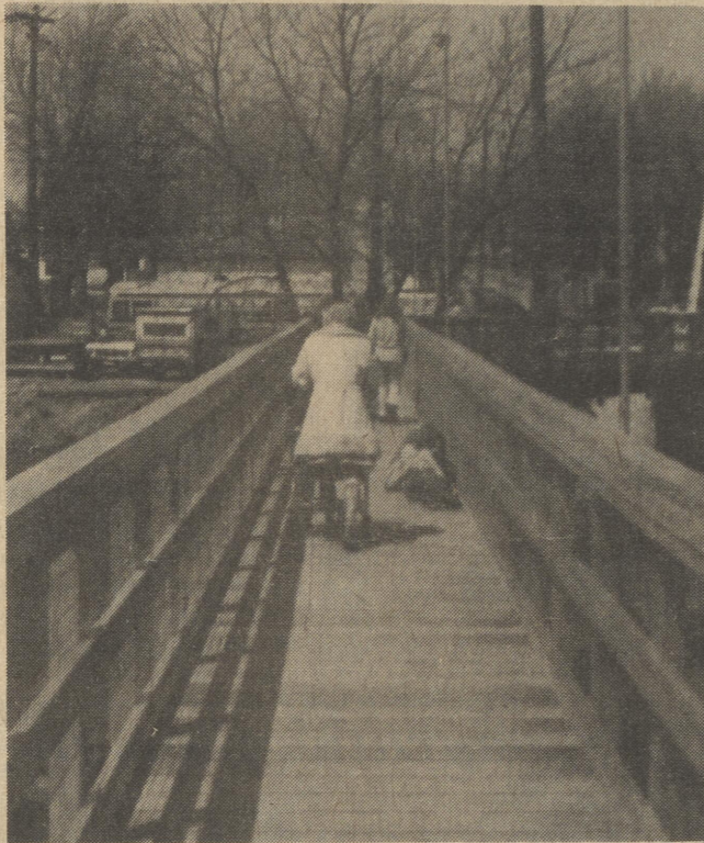
As the State Highway Administration of Maryland promised the footbridge for pedestrian traffic over the fallen Choptank River Bridge has opened within two weeks of the collapse of the old bridge. On Tuesday several people were taking advantage of the footbridge and according to one of the workers, "There is always a crowd of people using the footbridge."
