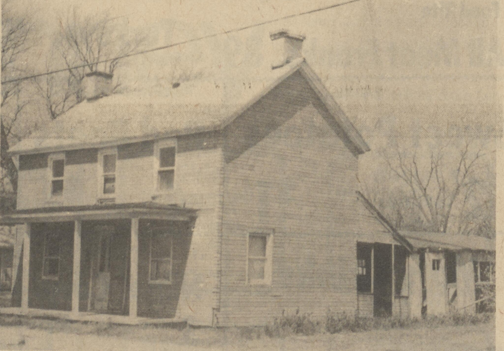
On Mechanic Street, this house on a Van Geisel property has been slated to be demolished.
