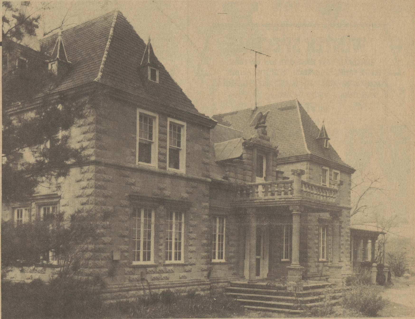
The Vogl House near Mastens Corner has been named to the National Register of Historic Places by the National Park Service. The blocks for the home were molded on the premises in a Sears Block Machine. Photo by Edward Heite
