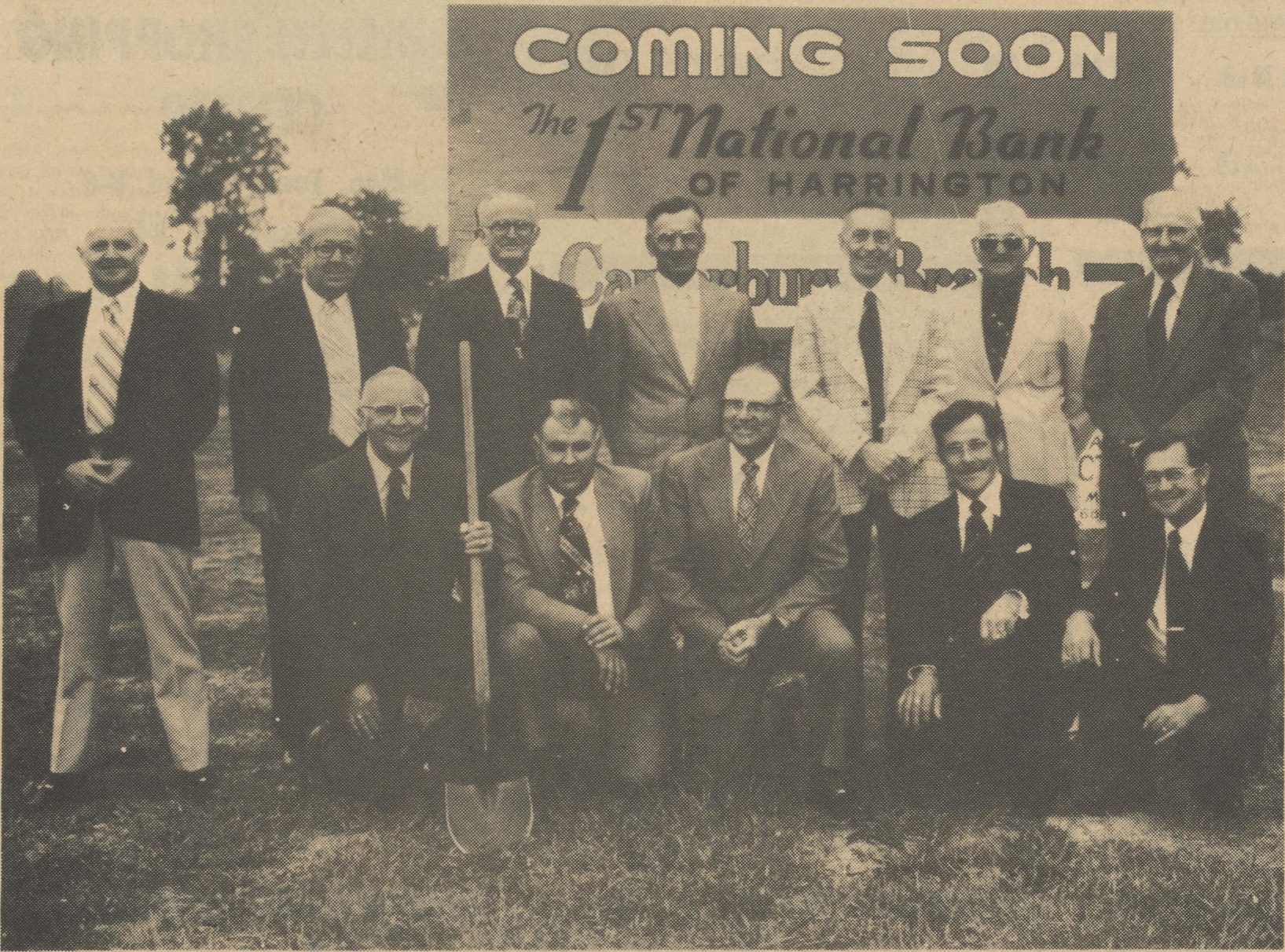
Officials of the First National Bank, Harrington, gathered at the site of the groundbreaking for the bank's first branch, to open in Canterbury sometime next spring.
