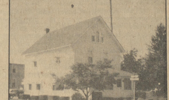
Harrington - 2 story frame, 3 brm. home in excellent condition. B.B. hot water heat, panelling throughout, carpeting throughout, garage. Priced for immediate sale and occupancy.
