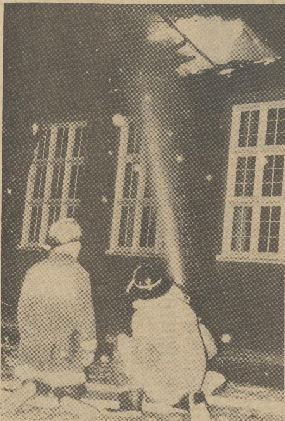
Fire at the Lake Forest East Elementary in Frederica originally broke out through the roof area. Above firefighters attempt to contain and control the blaze in hope it wouldn't spread too far.
