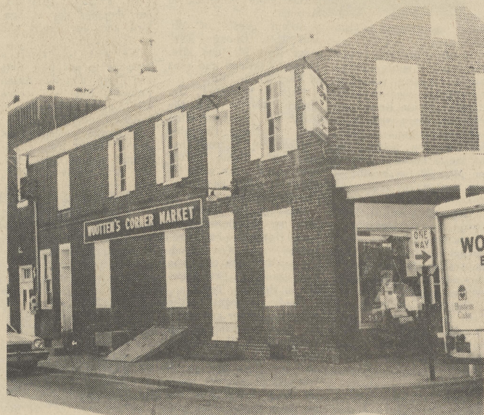
Wootens Grocery Store has been a Corner store for as long as anyone can remember. The two street fronts are laid in Flemish bond.
