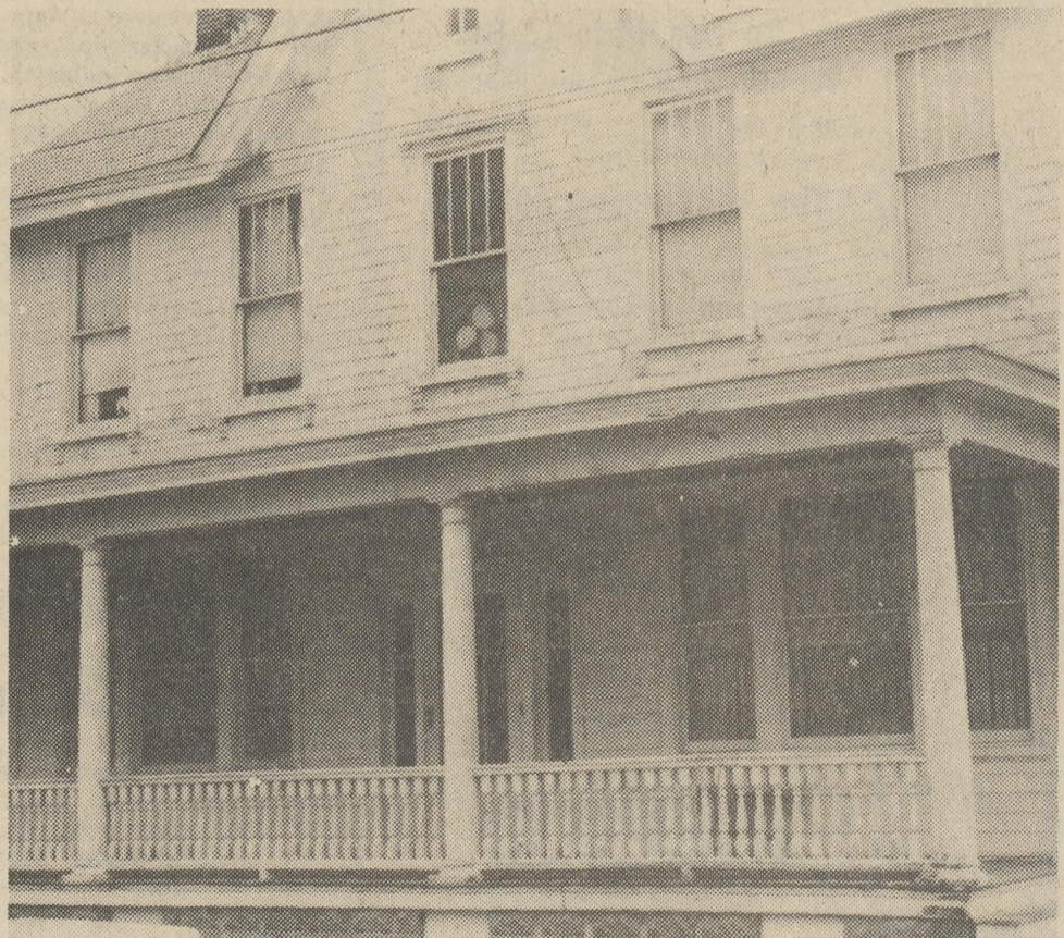
The Smithers House, south of the bank parking lot, is a large Victorian frame house. It was extensively remodeled in 1917.
