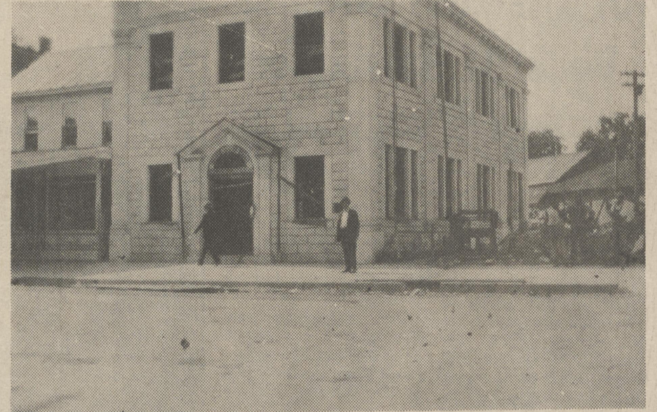
Work begins on the new bank building. [Above] Picture was taken August 13, 1927. [Lower] According to the records September 20, 1927. The outside was completed. Benaiah Tharp is seen standing at the corner of the building. At a later date the vacant lot to the right of the Bank was opened up for Fleming Street.
