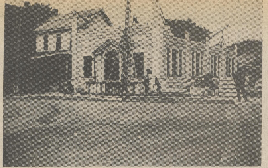
Work begins on the new bank building. Picture was taken August 13, 1927.
