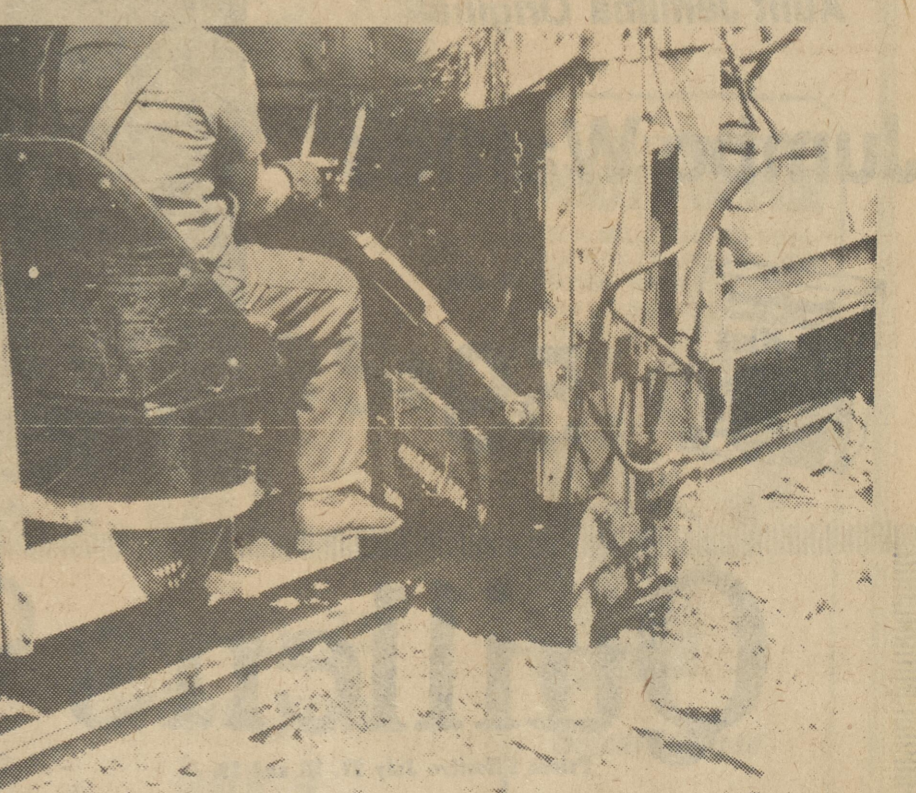
to the final step of driving the spikes.
