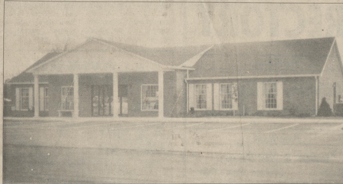
1st National Bank of Harrington at Canterbury.
