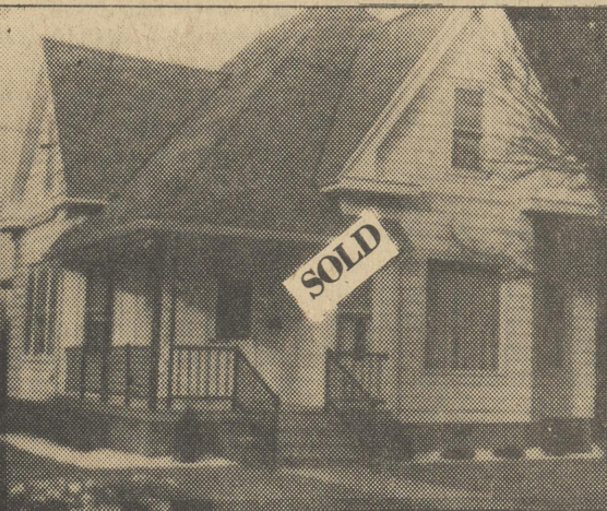
New Listing - Two Brm. home on Center St. Excellent cond. New carpeting, alum. siding - large rooms. Asking in low $30's. Also single car garage expandable 2nd floor.
