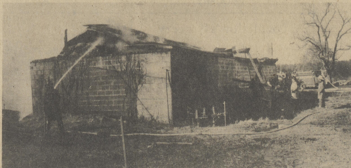
A fire on the Whiteleysburg Road on Monday morning left David Marvil without a straw barn. The fire started with an electrical short and quickly spread throughout the structure. The Harrington and Houston Volunteer Fire Companies responded and put out the blaze.
