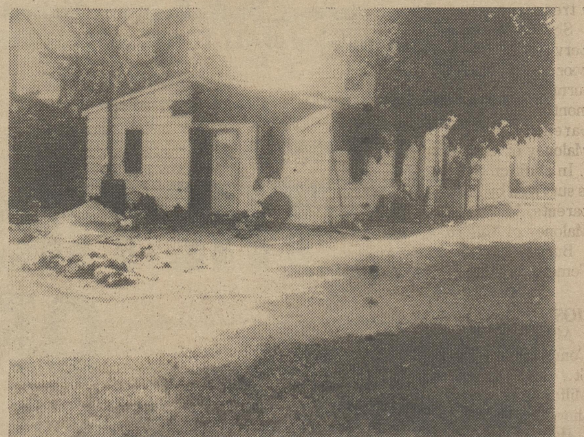
Harrington Volunteer Firemen responded to a fire on Weiner Avenue on Monday around 6 p.m. It was the former office of Dr. Addis. It is believed the cause was electrical possibly starting from a faulty motor in an electric fan. No one was in the house at the time of the fire.
