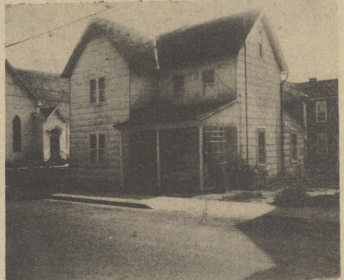
Two bedrm two story home in Harrington on a corner lot. Mostly renovated. New heating, plumbing and electrical systems.
