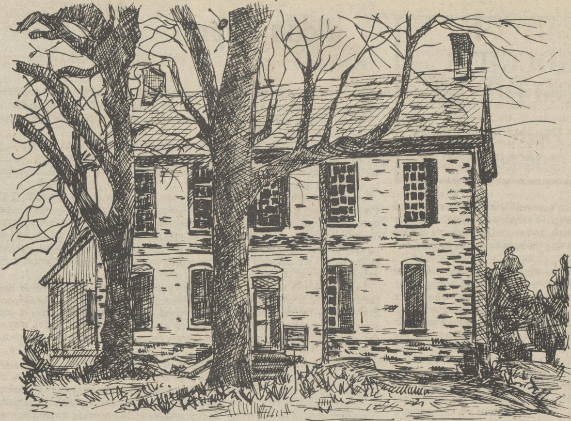
The Peter Lowber House and more recently called The Hathorn-Betts Home in Frederica is the sketch this week by Gretchen Banks. The house dates back to the mid-18th century, and is currently under construction by Simpson Lumber in Camden
