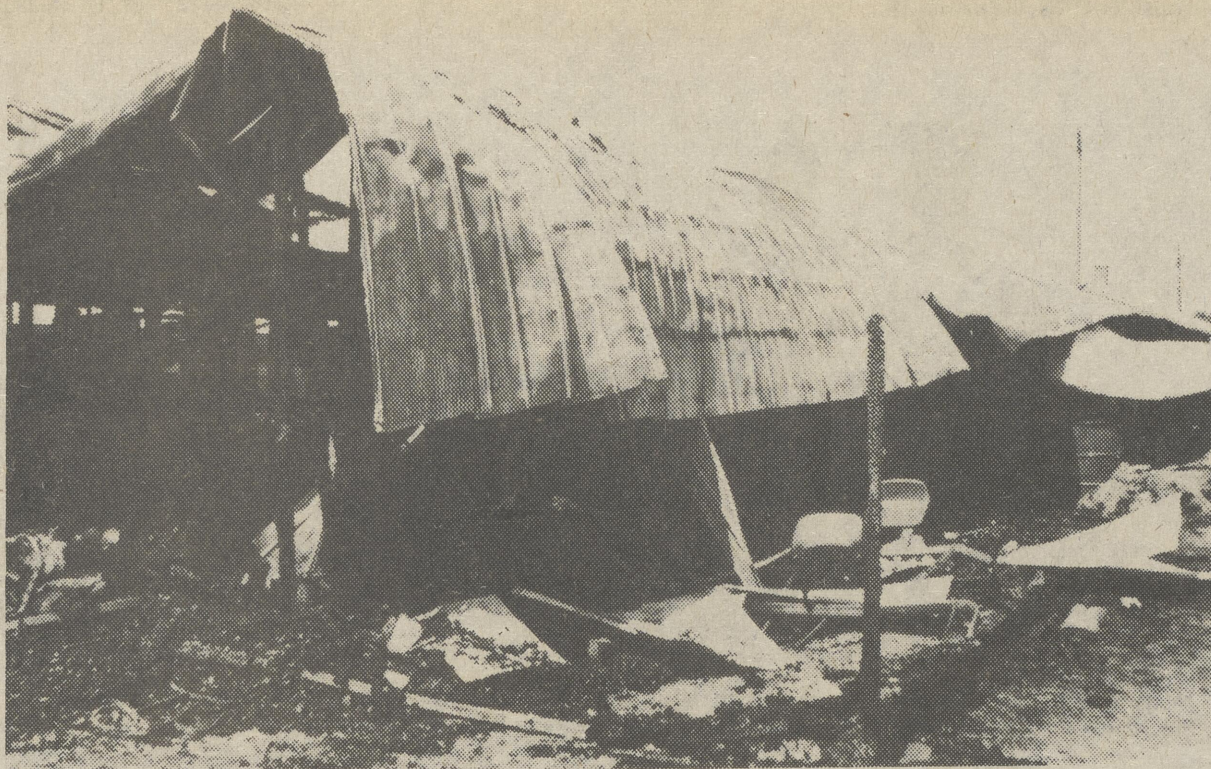
This was all that remained of a barn and eleven horses after a disastrous fire at Harrington Raceway Tuesday morning. Harrington, Farmington and Houston Fire Companies responded, while Milford, Felton and Greenwood were on standby duty.
