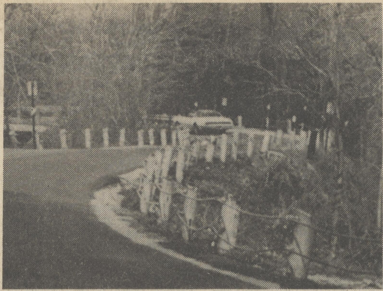
BEFORE --- This curve on the Andrews Lake Road was deemed a safety hazard until-----
