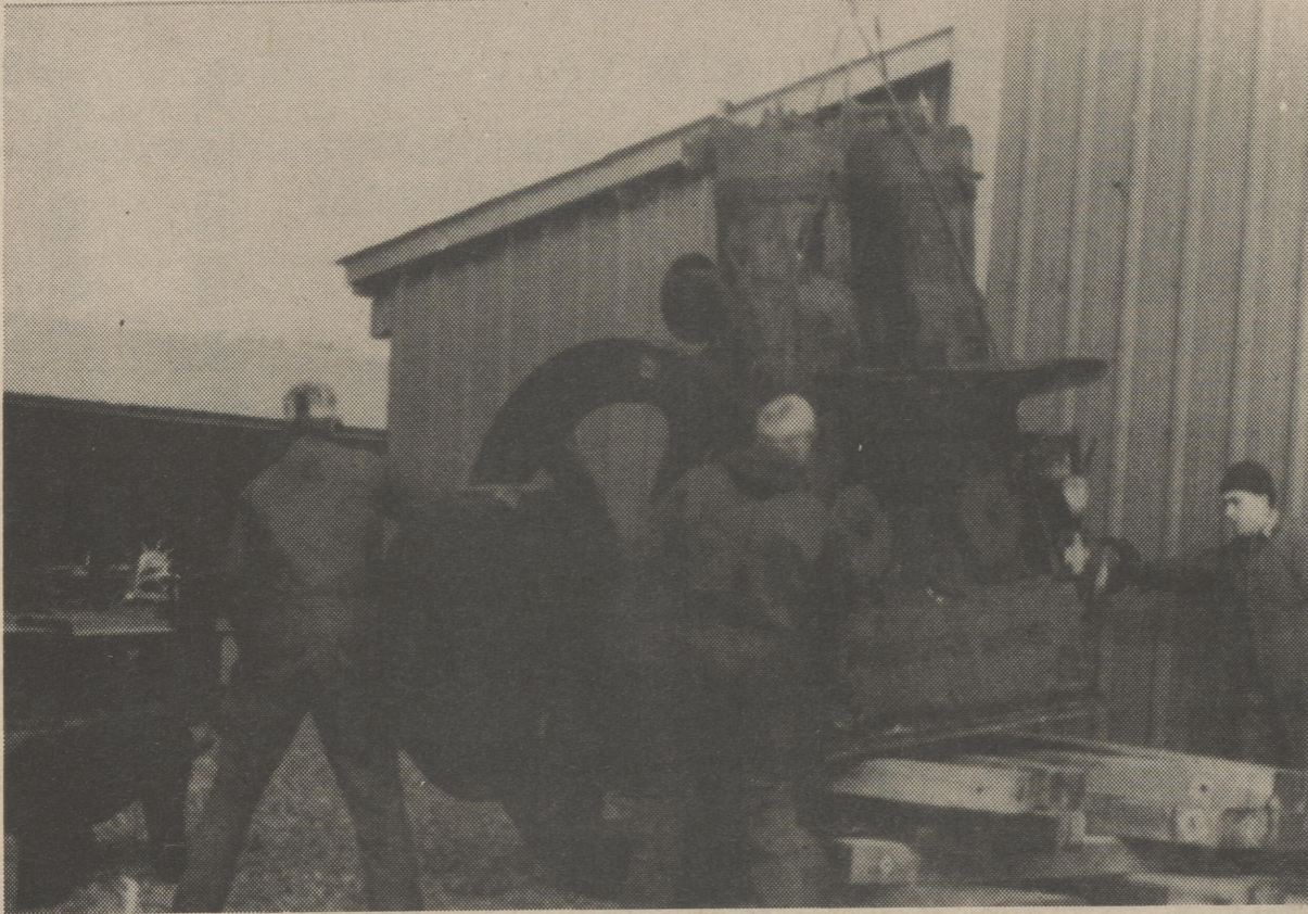
"Easy does it." - Walter Messick and crew guide this massive Fairbanks-Morse engine into place at the rear of Messick's Antique Museum. The 9 ton, 80 hp gasoline engine was lifted from its flatbed trailer with the help of a crane from First State Crane Service in Frederica. Purchased in Kenton last week, it is the latest addition to the Messick Antique Collection.
