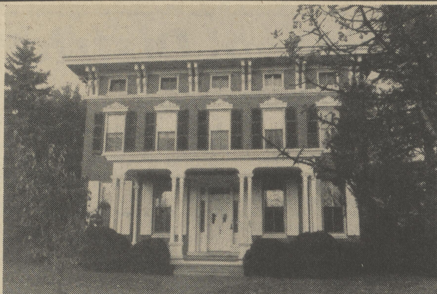
The Miller-Polk House is the main one of three adjacent houses built by the Polk family (leading wheat merchants) during the mid-1800's. The house was designed by Samuel Sloan of Philadelphia and is the home of Dr. Marian Miller. This house was on tour in 1983.
