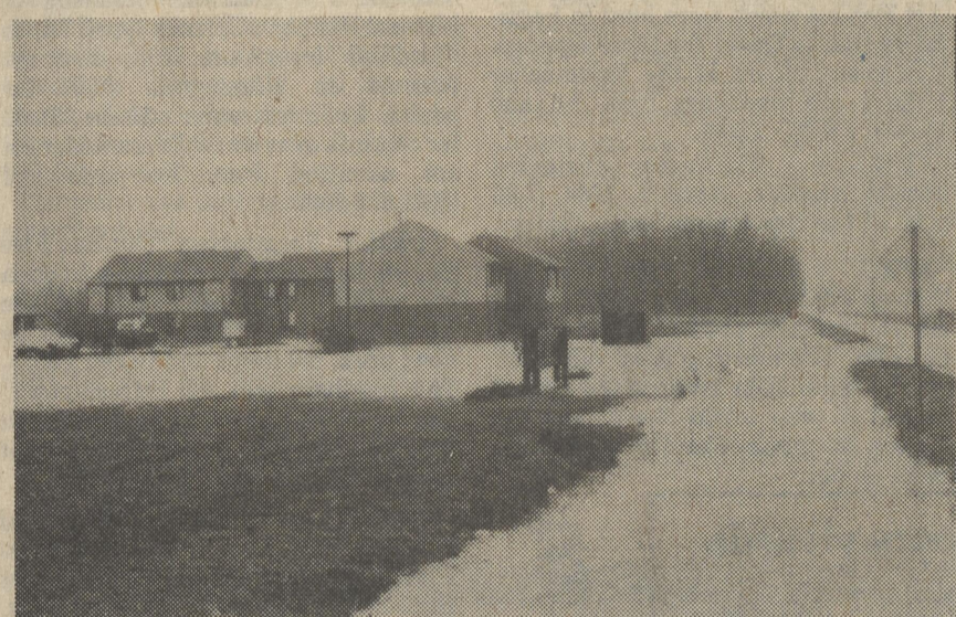
The storm on Thursday caused flooding at Clark's Corner project. Photo by HGF
