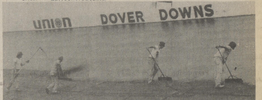
DOVER, DE — the Dover Downs International Speedway "Goo Crew" at work applying 4500 gallons of asphalt sealer to the racing surface. The "Goo" will get its first workout during the May 19, 1985 Budweiser 500 at the high banked Delaware superspeedway. (Photo by Jack Olenik)
