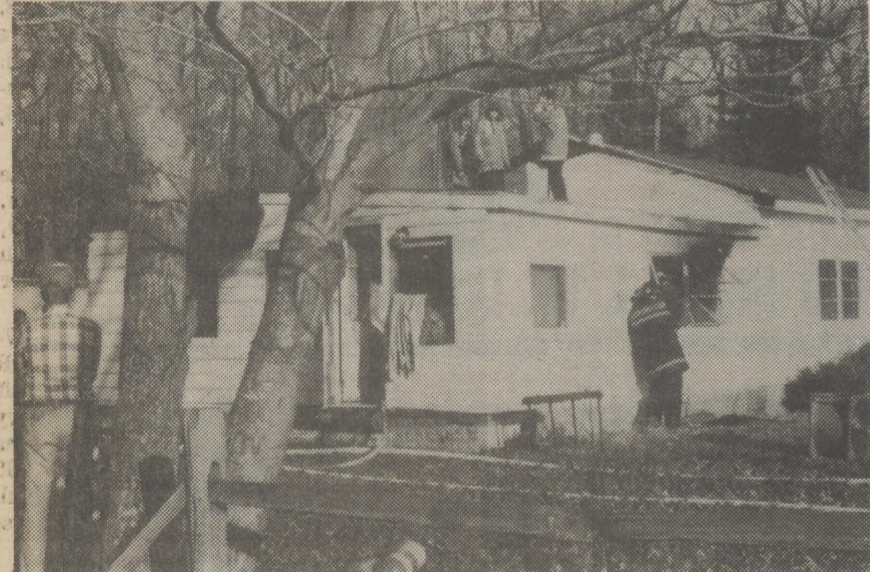
This house and trailer combination living quarters caught fire on Thursday, Dec. 20. The house is located on County road 441 South of Farmington. The Greenwood and Farmington Vol. Fire Companies responded with Harrington backing up Farmington. Damages were extensive but there were no injuries. Photo by HGF
