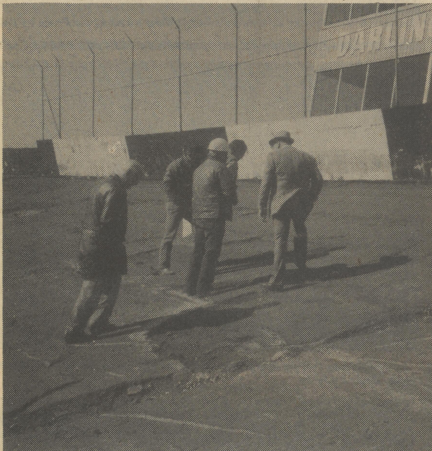
DOWN TO THE DIRT — Darlington raceway officials take a look at the asphalt in the first turn, some of which was three feet deep. It was decided to "plow" up the first turn and put down new asphalt before the running of the Dixie Cup 200, Saturday, April 13th and the Transouth 500, April 14th at the track the drivers call "too tough to tame."
