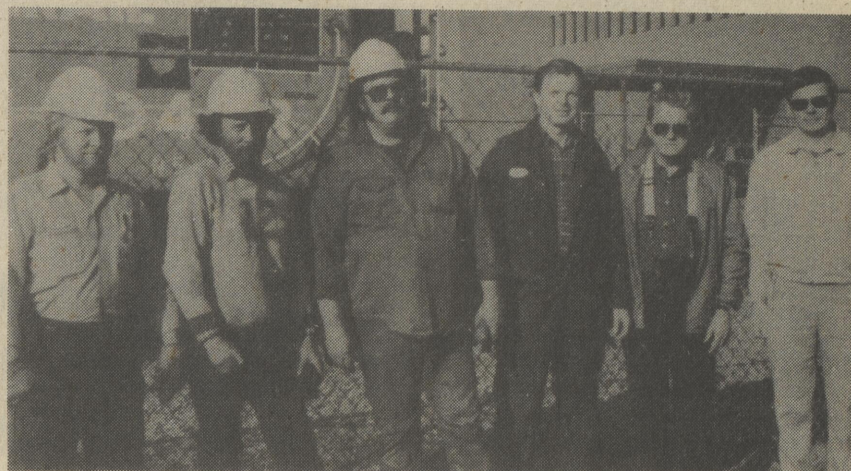
The Harrington Historical Society wishes to recognize the following railroad crew who directed the operations of installing the caboose on the museum grounds. They are, left to right, Ernie McCarter, chief of the project; Ron Muncey, Dave Kennedy, Gerald Shank, Donnie Jester, of the Harrington Historical Society and Jerry Hayman, also of the Society. The latter two coordinated the efforts to get the caboose.
