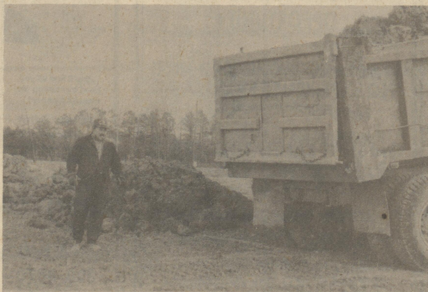
Georgetown Speedway Director Tony Donofrio supervises the dumping of a portion of the over 1000 tons of new clay brought in for the track surface on January 15th. An estimated 12 inches of new surface are added to the turns. Photo by Jim Ritchie. D&L Photos
