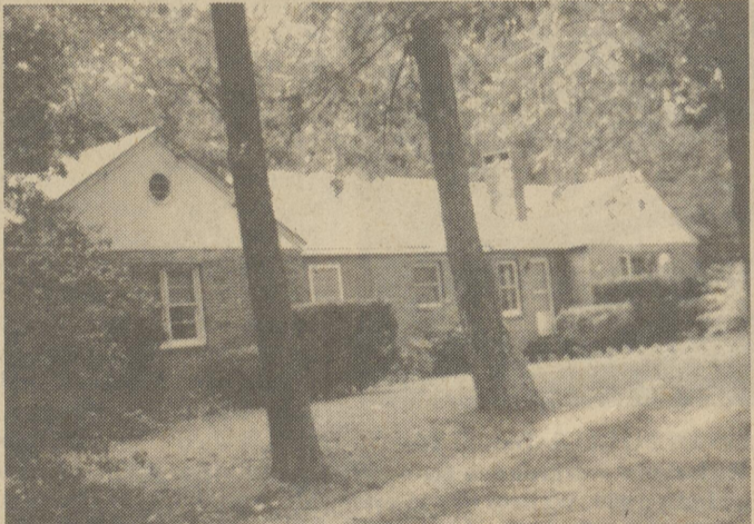
CUSTOM BUILT BRICK RANCHER on 5 acres, full basement, double garage. Lovely home. Call for appointment- $110,000.
