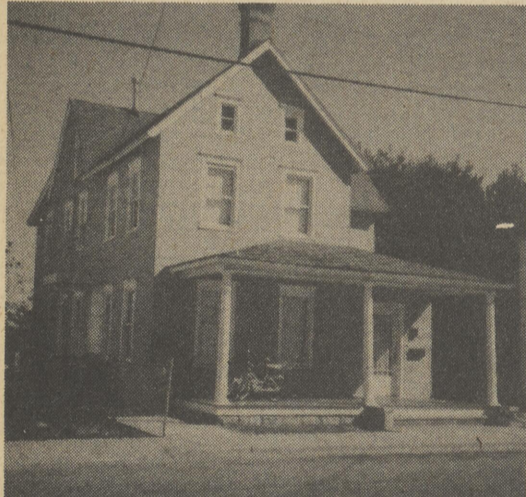
TWO FOR THE PRICE OF ONE—Two one bedroom apartments—New PVC plumbing, updated electrical, insulated. $40,000.
