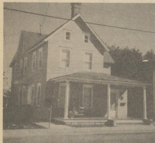
TWO FOR THE PRICE OF ONE -Two one bedroom apartments-New PVC-plumbing, updated electrical, insulated. $40,000.
