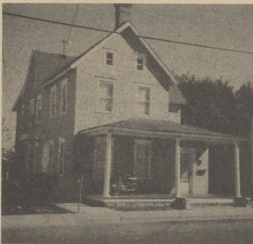
TWO FOR THE PRICE OF ONE —Two one bedroom apartments—New PVC plumbing, updated electrical, insulated. $40,000.
