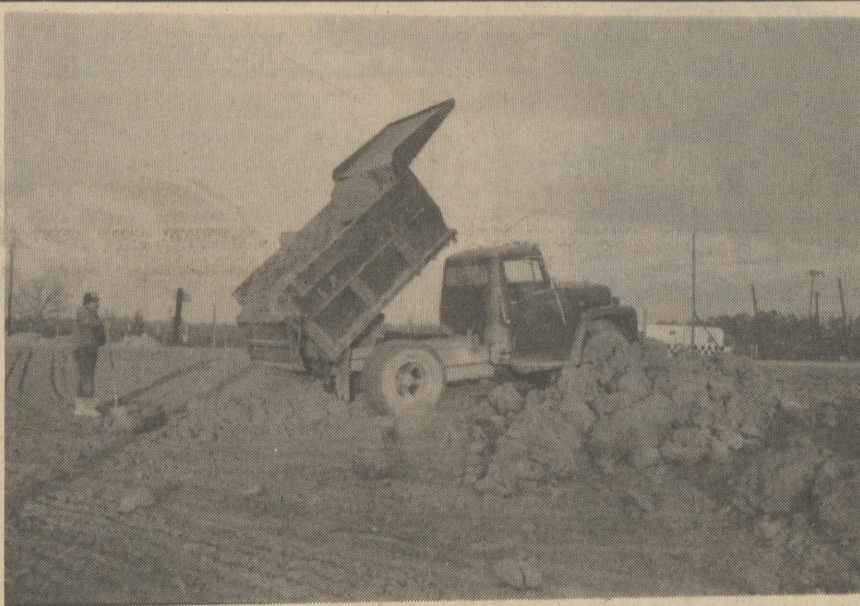
Georgetown Speedway Director, Tony Donofrio, supervises the dumping of one load of the nearly 1800 tons of new clay added to the track surface in mid-January. Photo by D & L Photos
