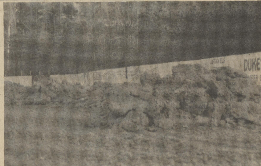
Shown is a portion of the nearly 1800 tons of new clay added to the Georgetown Speedway track surface in mid-January. It should make for some super racing in 1987! Photo by D & L Photos
