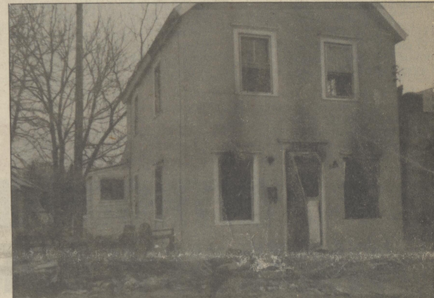
Late Monday afternoon fire destroyed this home at 6 West Liberty Street in Harrington. Members of the Lake Forest Ministerium are seeking the names of the occupants of the house in order to find them shelter. Photo by HGF
