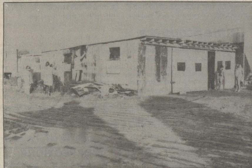
A fire broke out in Sam Powell's pig building Tuesday morning. Harrington Fire Company responded and extinguished the fire. Damages were minor. Photo by HGF.
