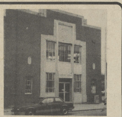
HARRINGTON —Located on Commerce Street, 2-story multi-purpose building, formerly a bank. Very well maintained. 5,000 square feet with elevator. $97,000.
