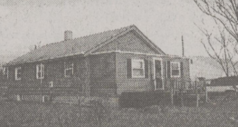
NEW LISTING! With lots of updates, incl. new roof, rep. windows & heater Cozy 2 BR, 1 bath ranch across from Shawnee Country Club. In process of remodeling. Modestly priced at $79,900. #1519.
